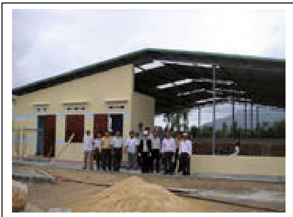
Compost plant constructed in Qui Nhon City of Vietnam
